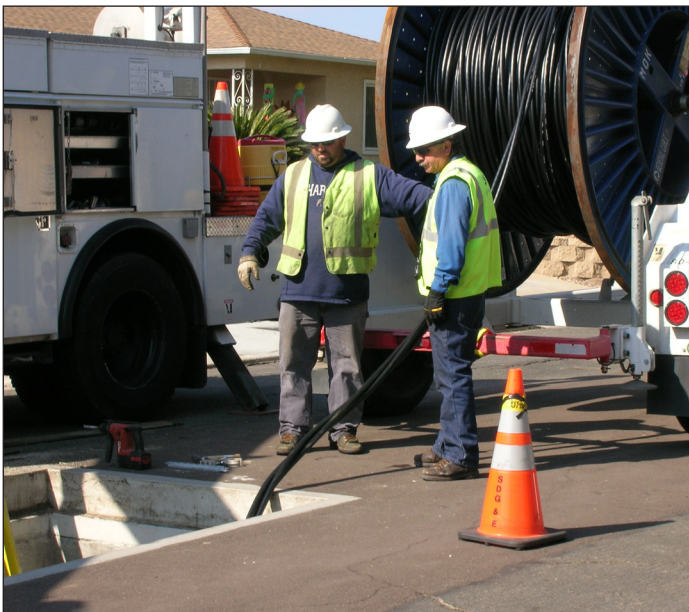
SDG&E crew members install cabling into one of their underground vaults.
